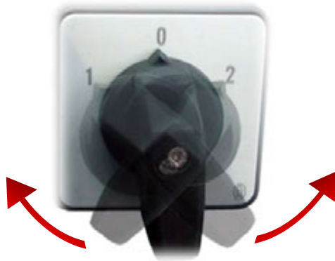
Figure 4. Main Control Switch
